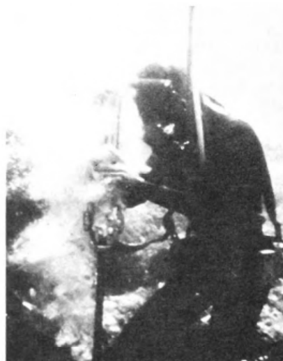
Divers used hand-held and tracked crawler pneumatic drills to drill dynamite holes for blasting out obstacles and leveling steep slopes along cable path. They also drilled holes in the rocky floor for placing U-bolt anchors to prevent cable motion and possible fatigue failure.
