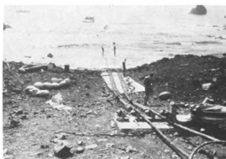
Installing cable protectors in the dry saved nearly one month for the operation as compared with conventional underwater method of installation.
